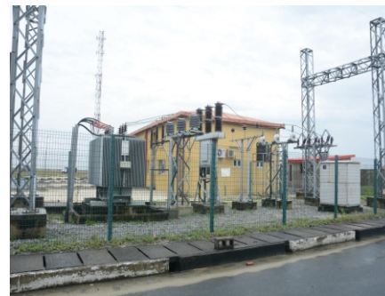
5 MVA TRANSFORMER INSTALLED AT THE SITE
